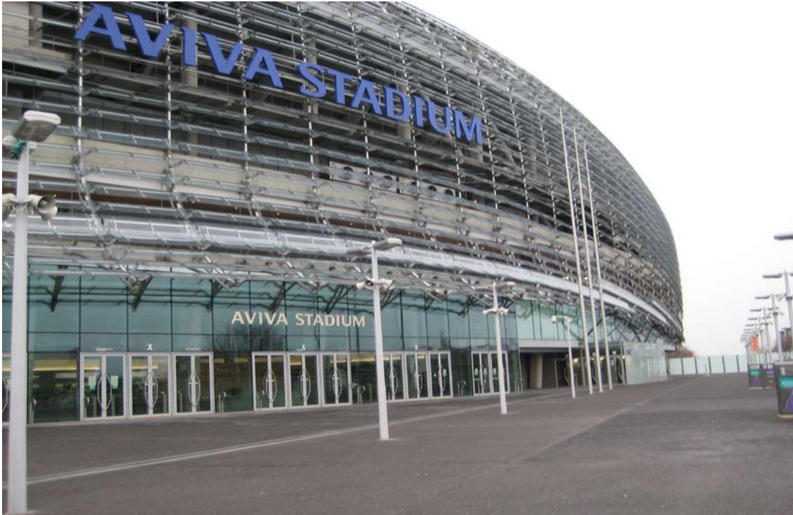
Completed construction of Aviva Stadium
